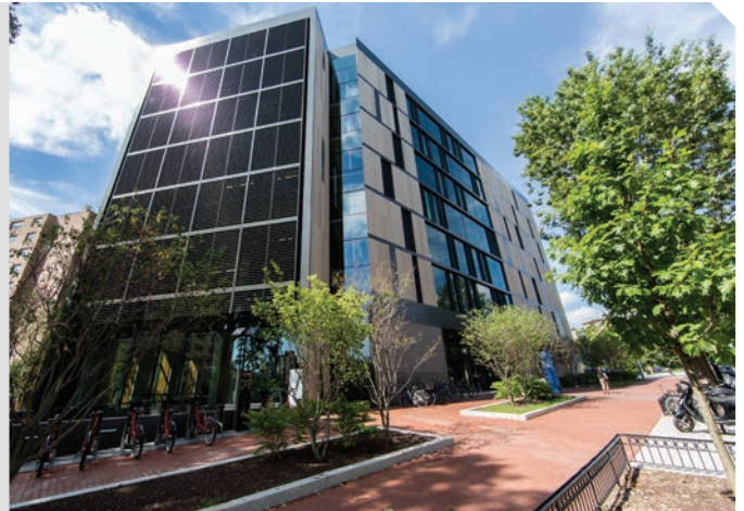
GW achieved its first LEED Platinum certification for the Milken Institute School of Public Health.
